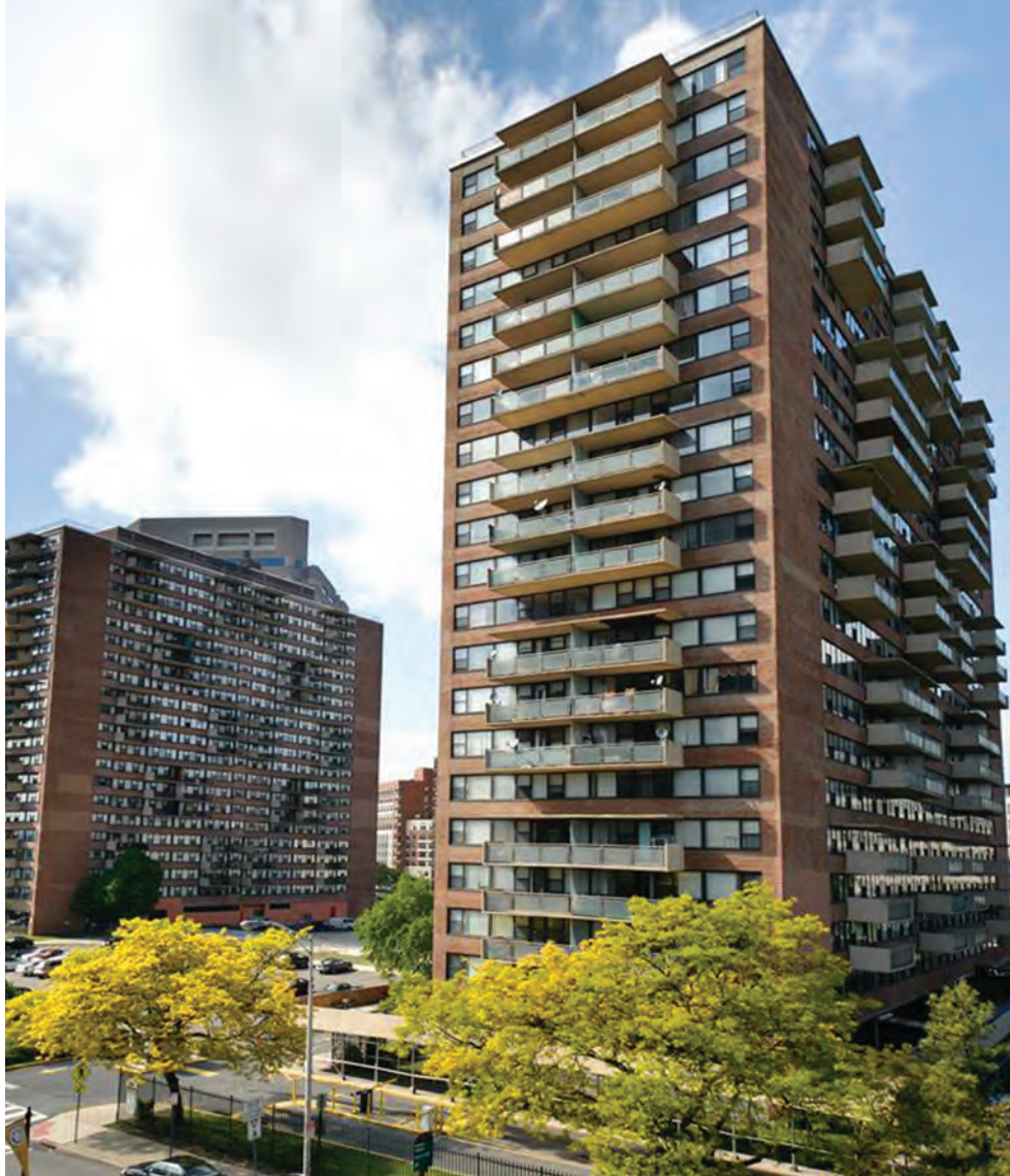
Excavation at Metropolis Towers was completed in June 2014 with continuous air-monitoring indicating quality was well within NJDEP standards.
